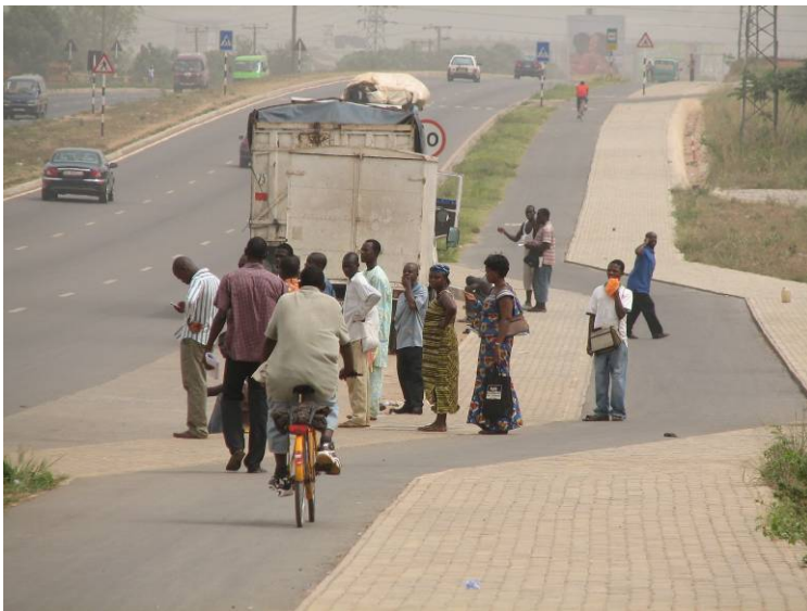
Separated motorway, bus stop, cycling lane and foot path, Accra Photo: L. Eickmans / Cycling out of Poverty
